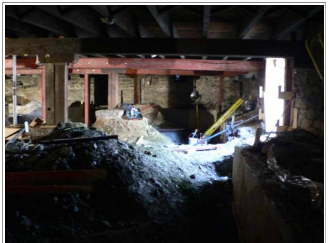
The excavation of the crypt with new steel girders in place.
